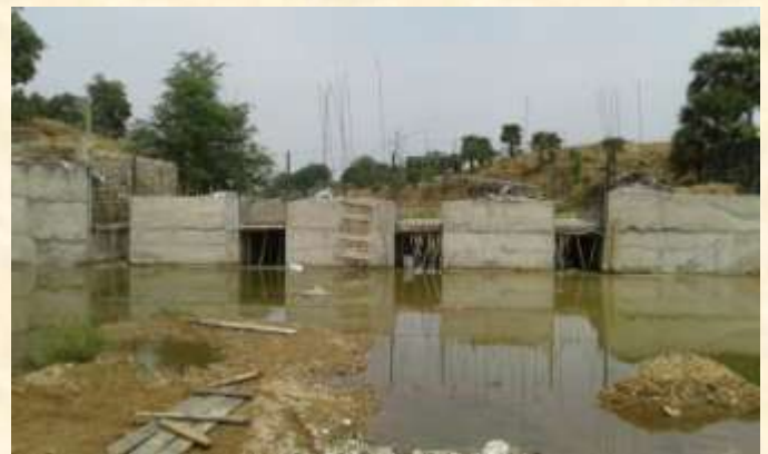
Check Dam at Dimdiha-Ghagra villages
