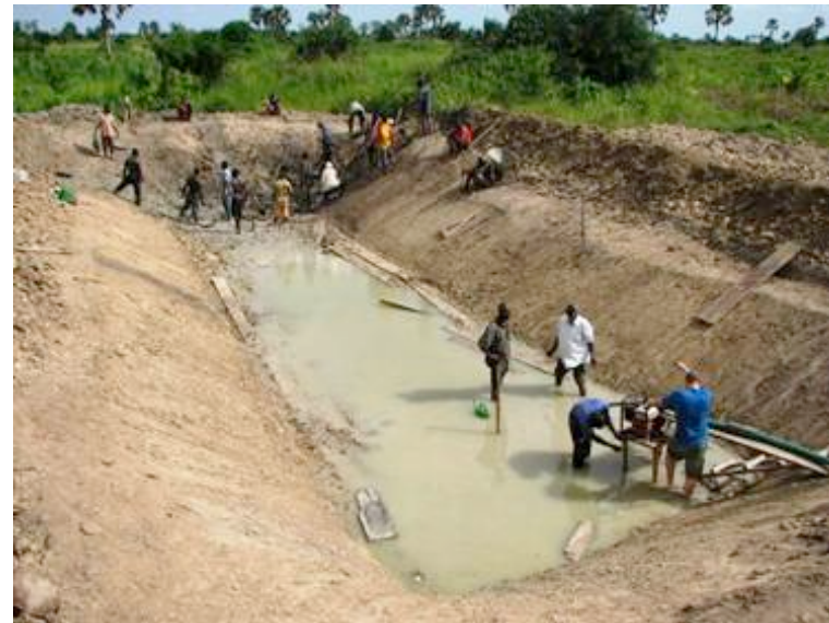
The drainage canal pit was dug by manual labour
