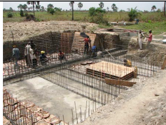
Starting the formwork after pouring foundation
